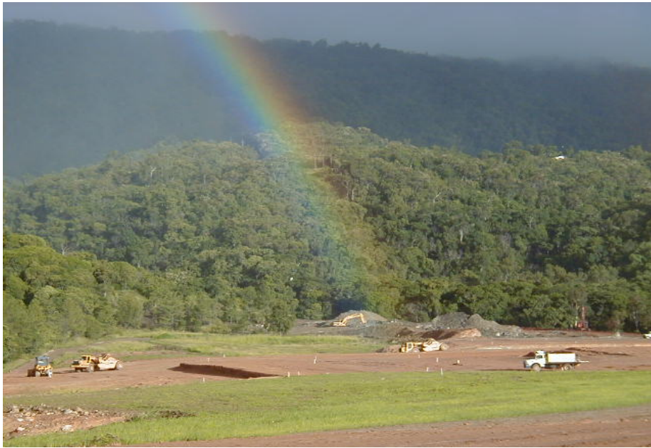
A view of Canopy's Edge during construction
